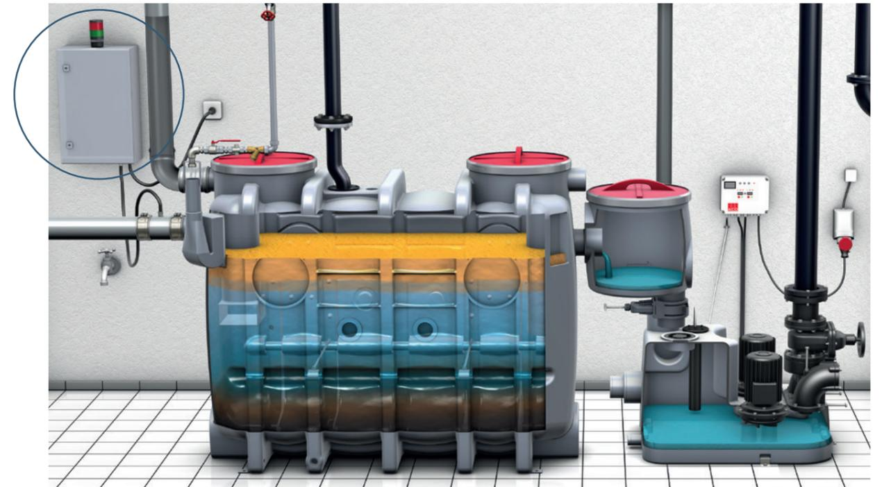
The ACO odour neutraliser significantly reduces the formation of noxious smells in all vent stacks and plant components.
