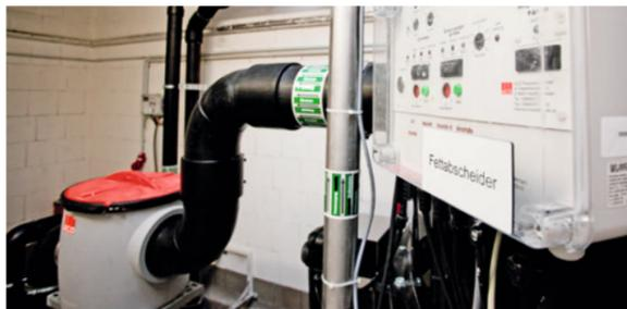
For operational reasons as well as due to local regulations, fatty waste water from commercial kitchens may not be discharged directly. ACO grease separators pre-treat the wastewater, which prevents the pipes connected to the drain from becoming greasy, thereby ensuring the operational safety of the kitchen.
